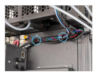
Insert the zip-tie through the metal cut-out and secure all cables. Do not overtighten the zip-tie. Cut the ends of the zip-ties.
